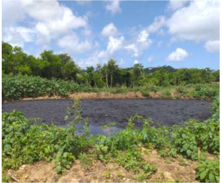
One out of the four affected pits with the Oil Sludge
