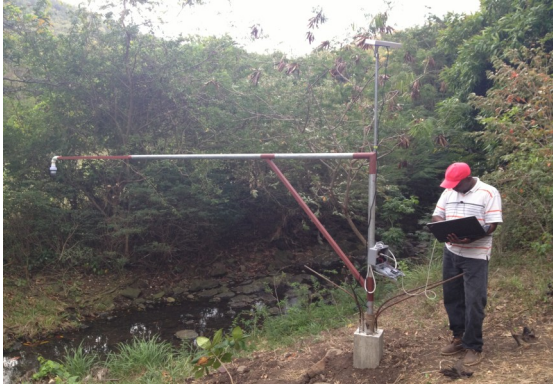
Water Level Sensor
