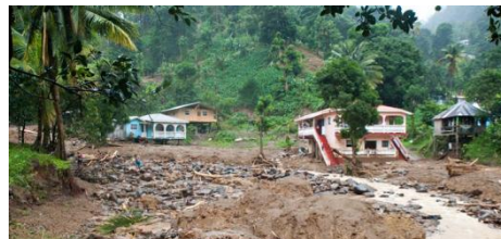
SILT AND DEBRIS DEPOSITION BY THE SOUFRIERE RIVER ALONG MAIN CHANNEL AT FOND ST JACQUES
