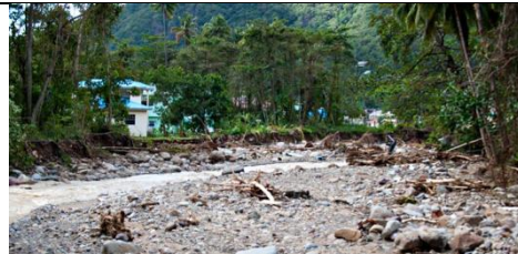
SILT AND DEBRIS IN THE MAIN CHANNEL DEPOSITED BY THE SOUFRIERE RIVER NEAR NEW DEVELOPMENT
