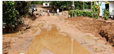
REMNANTS OF REPORTED 5 FEET FLOOD WATERS AT MARC AND SILT DEPOSITION ALONG DRAINS AND ROADWAYS
