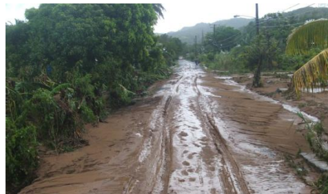
SILT DEPOSITED BY THE DENNERT RIVER NEAR MOLE ROAD
