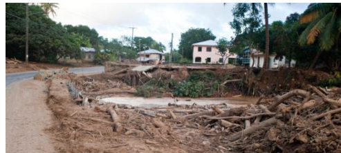
SILTATION AND DEBRIS DEPOSITION BY THE FOND DOR RIVER NEAR THE GRANDE RIVIERE BRIDGE
