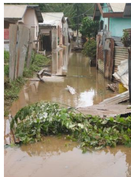
FLOODING AND SILTATION IN DENNERY OFF THE MAIN STREET
