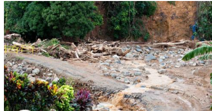
SILT AND DEBRIS DEPOSITION ALONG THE MAIN RIVER CHANNEL OF THE MARC RIVER AT MARC BRIDGE
