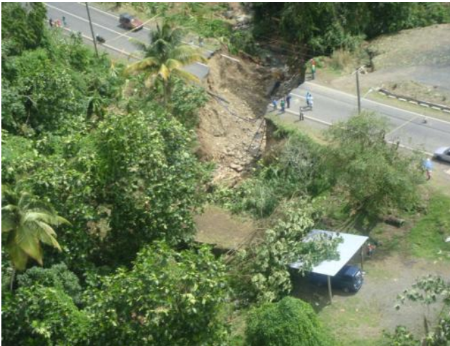
Figure 5: Destroyed road infrastructure
